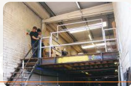
Figure 4 Fabrication of an up and over handrail
